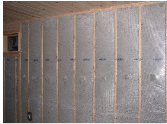
Celulose insulation, as delivered, and packed in wall behind a vapor barrier
