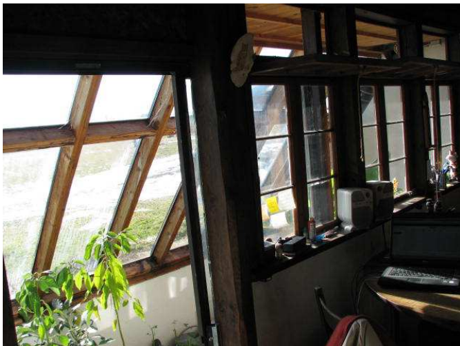
^ Heat distribution openings between greenhouse and kitchen. Movable insulation >
