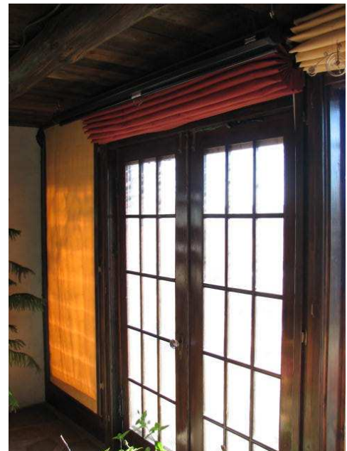
^ Heat distribution openings between greenhouse and kitchen. Movable insulation >
