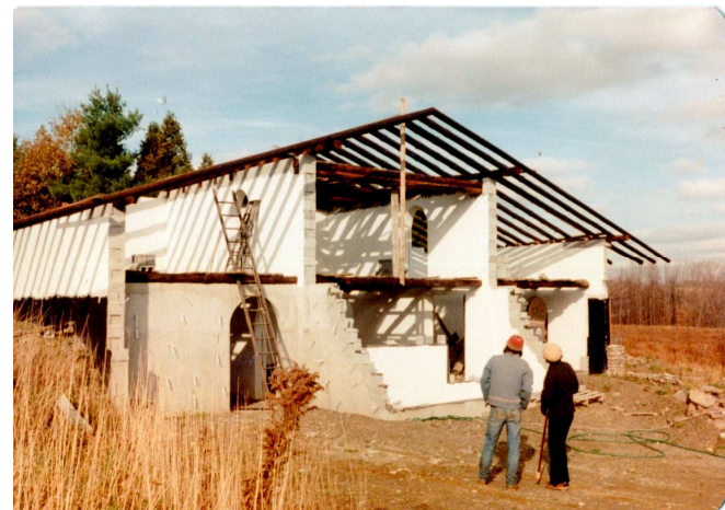
Dry-laid block and bonding cement make strong walls fast
