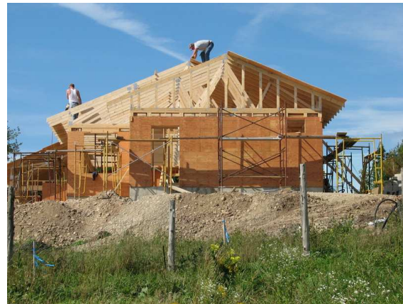
The raised truss design
