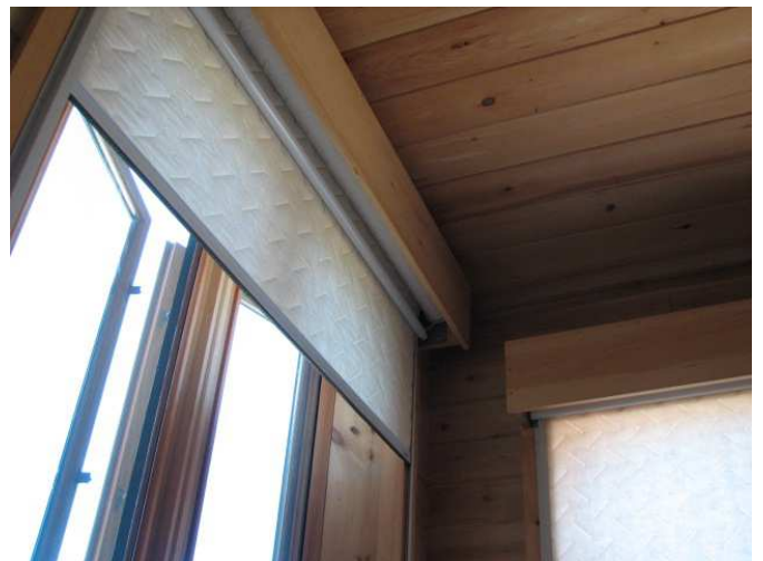
Movable insulation - shutters and quilts on rollers
