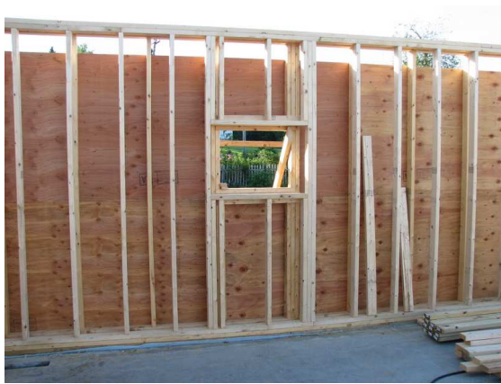
The double-walled frame
