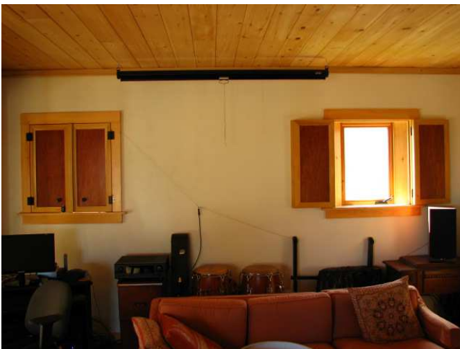
Movable insulation - shutters and quilts on rollers
